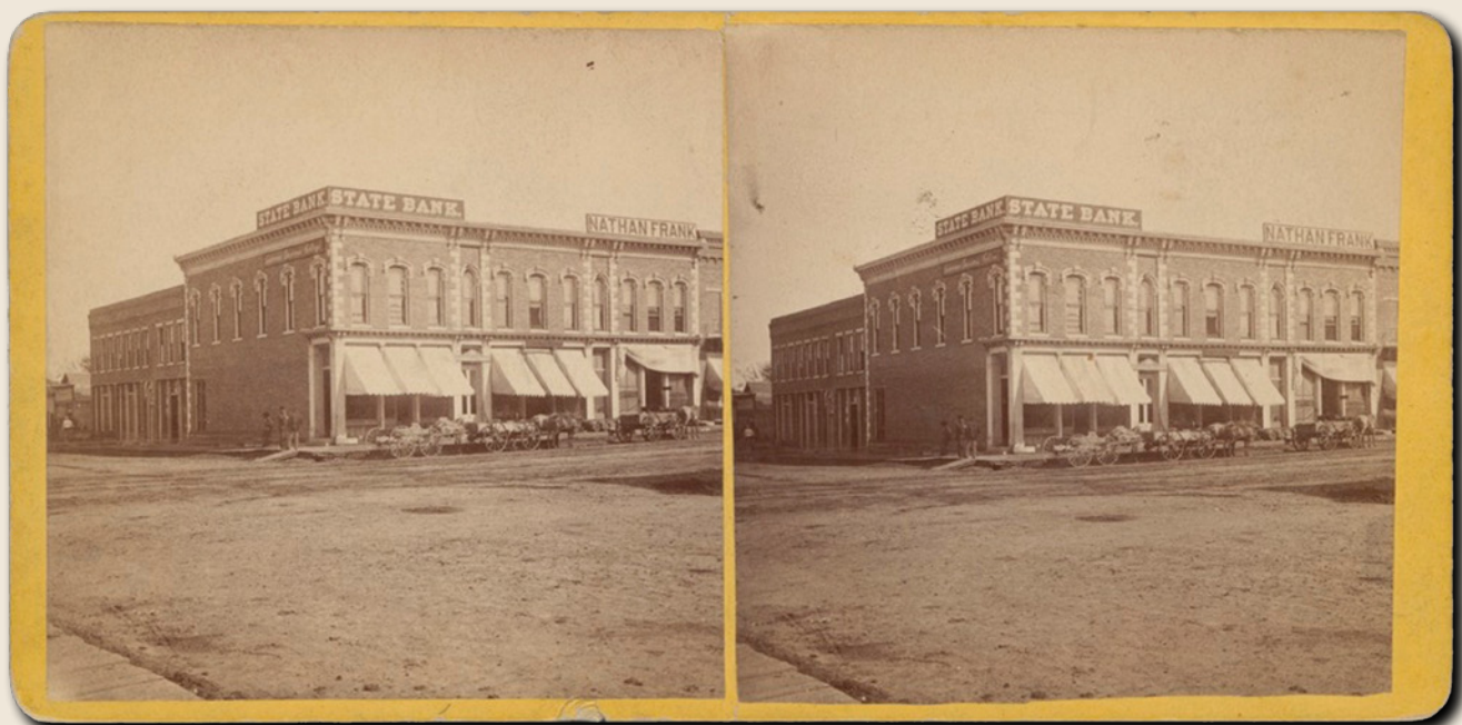
Business buildings on Massachusetts Street in Lawrence, Kansas. Signs for the State Bank and Nathan Frank, a wholesale grocer, are visible.
