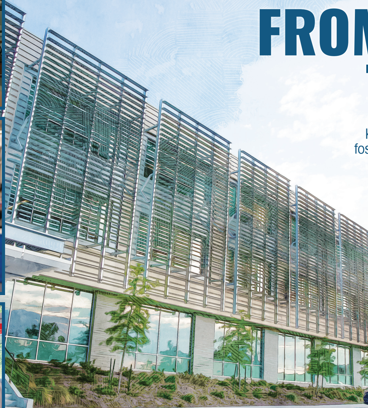
Background: The Phase 3 building at KU IP
