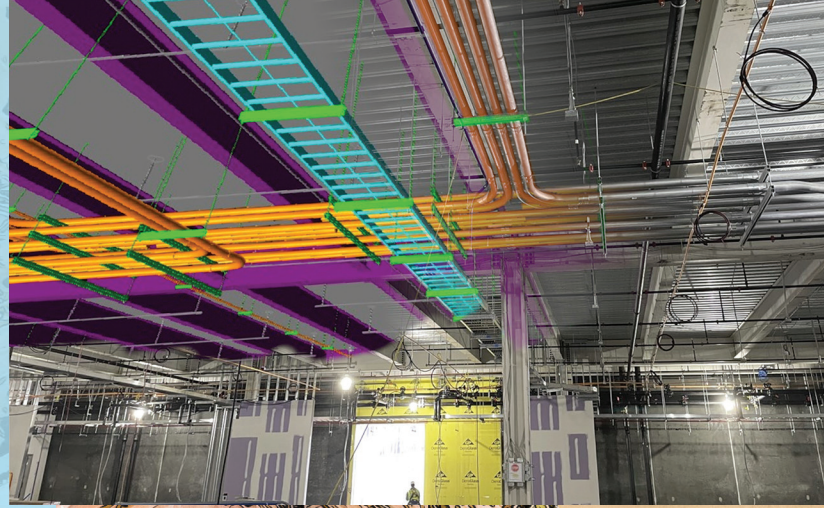
Michael Munson (right) and Heath Robertson (left) discuss layout options for an electrical room at a large corporate campus in Bentonville, AR
